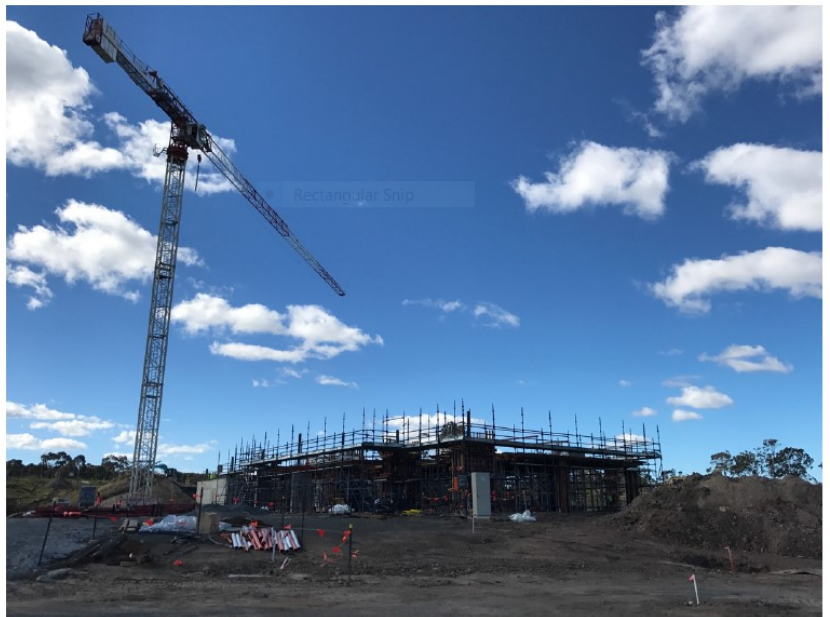
First floor slab formwork installation – Front plaza area – 04.08.17
