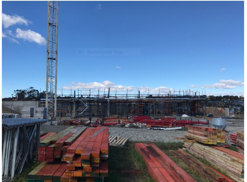
First floor slab formwork installation & retaining wall construction – northern site area – 04.08.17
