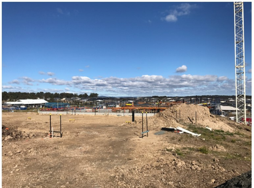
First floor slab detail cut and preparation – civic hub area – 04.08.17
